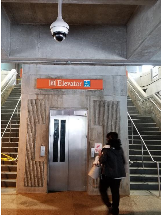
Increased CCTV Coverage Stations
